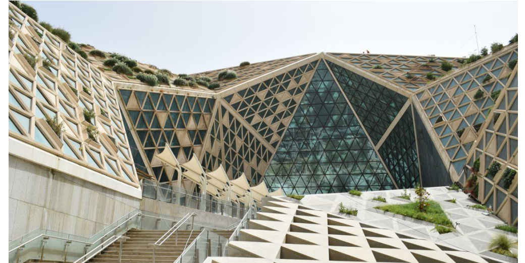
KAFD Conference Center 10,000 m 2
